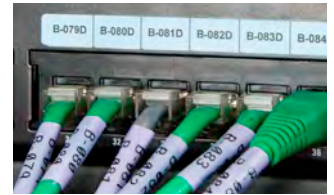
Patch Panel Labels
