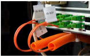
Fiber Optic Cable Markers
